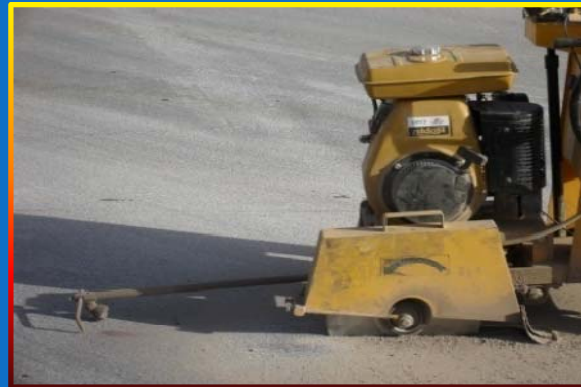
ASPHALT CUTTING
