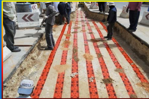
WARNING TAPE LAYING
