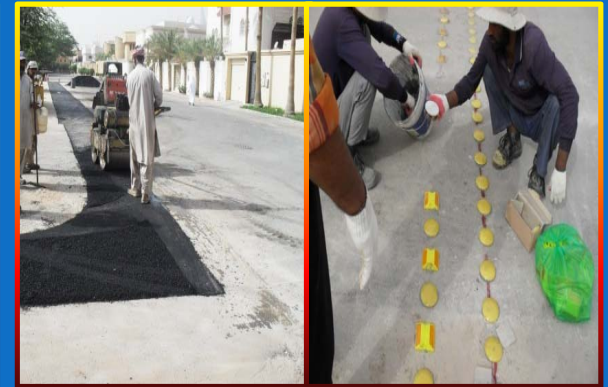
ASPHALTING/CAT EYE FIXING
