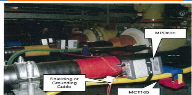
MPD 600 & HFCT INSTALLED AT A TYPICAL CABLE INSTALLATION LINK BOX
